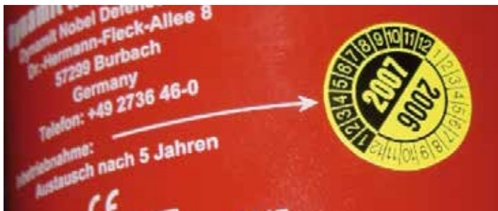
Fig 6: Affixing of the commissioning label
